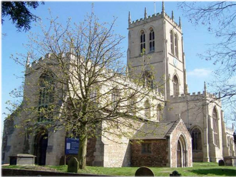
The Parish Church of St Lawrence, Hatfield
